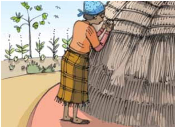
Figure 5: The framework is covered with grass.
